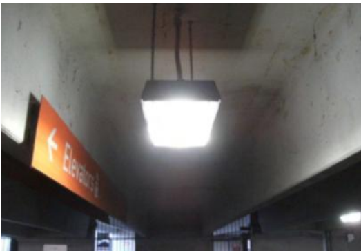
LED lighting retrofit at Lily Garage
