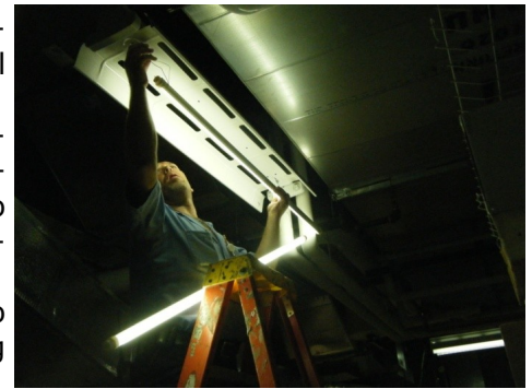
A mechanic inserts a new LED lamp into an existing fixture in a storage area
