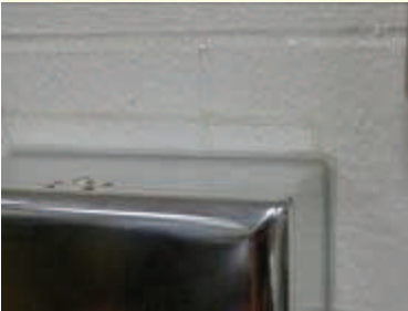
Caulking around a wall-mounted paper towel dispenser
