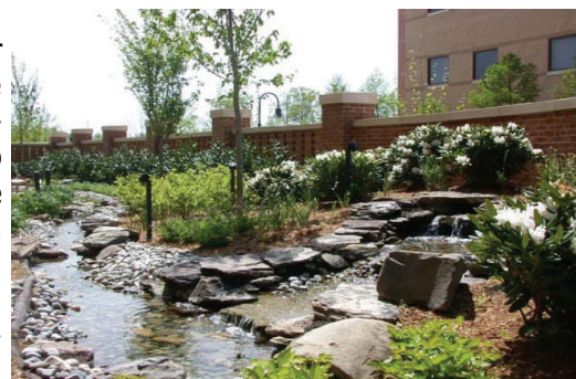
Step ponds have been designed to treat storm water runoff
